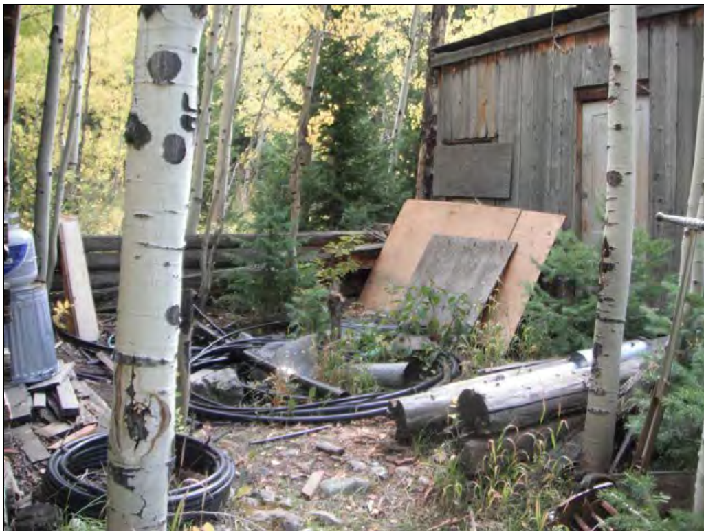
5GN6530 – Edgerton Cabin. View of the "backyard" showing the relationship of the east stretch of the log fence with the shed. View southeast. (Roll 19-261, image 132, 09/27/2019)
