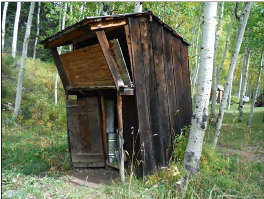
5GN6535 – Melton House. View of the shed. View northeast. (Roll 19-259, image 529, 09/26/2019)
