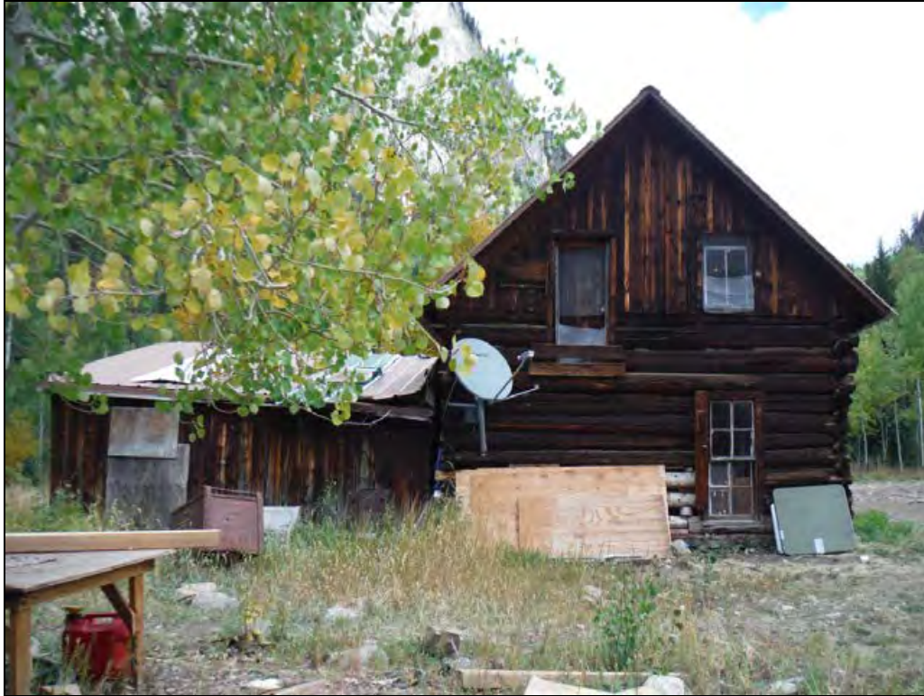
5GN6528 – General Store. View of south elevation. View north. (Roll 19-260, image 723, 09/27/2019)
