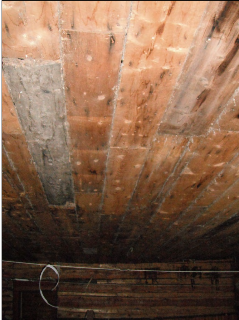
5GN6527 – Crystal Club. Interior, view of the ceiling of the main ground floor room in the original building. View east/up. (Roll 19-262, image 279, 09/27/2019)
