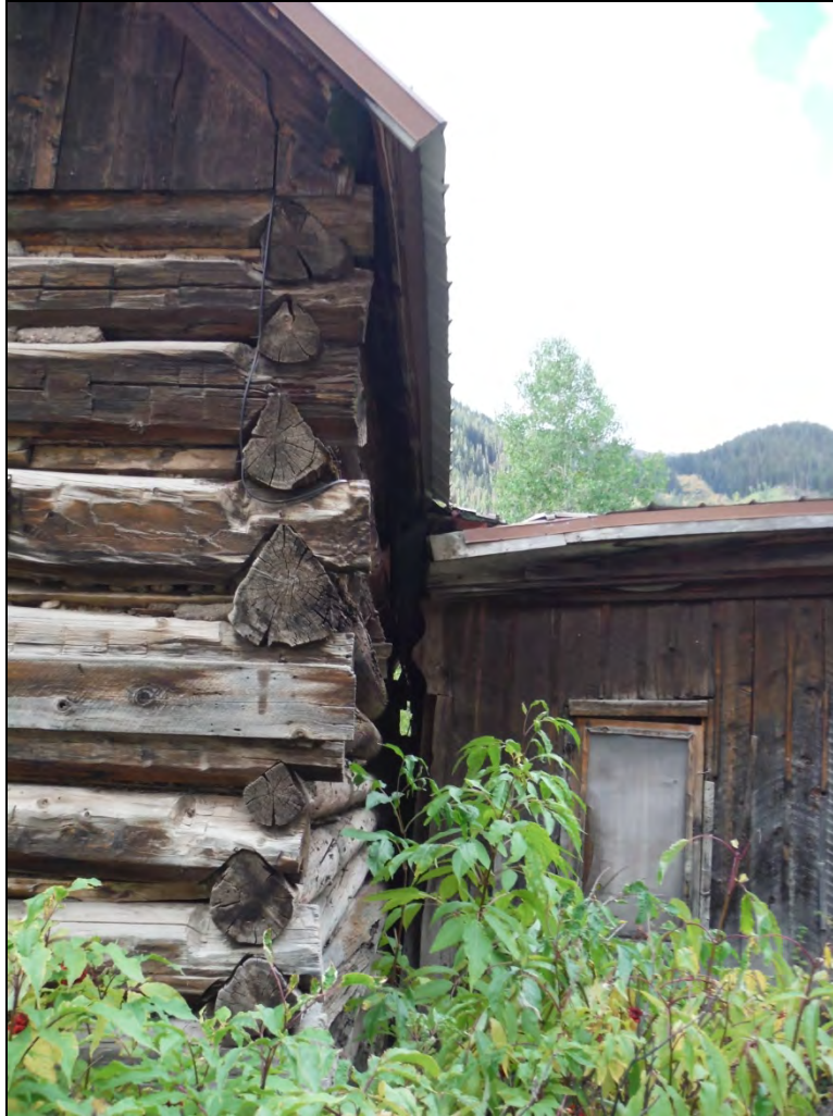
5GN6528 – General Store. Detail of steeple log notching on northwest corner. View south. (Roll 19-260, image 709, 09/27/2019)
