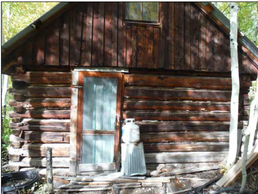
5GN6530 – Edgerton Cabin. View of south elevation. View north. (Roll 19-259, image 595, 09/26/2019)
