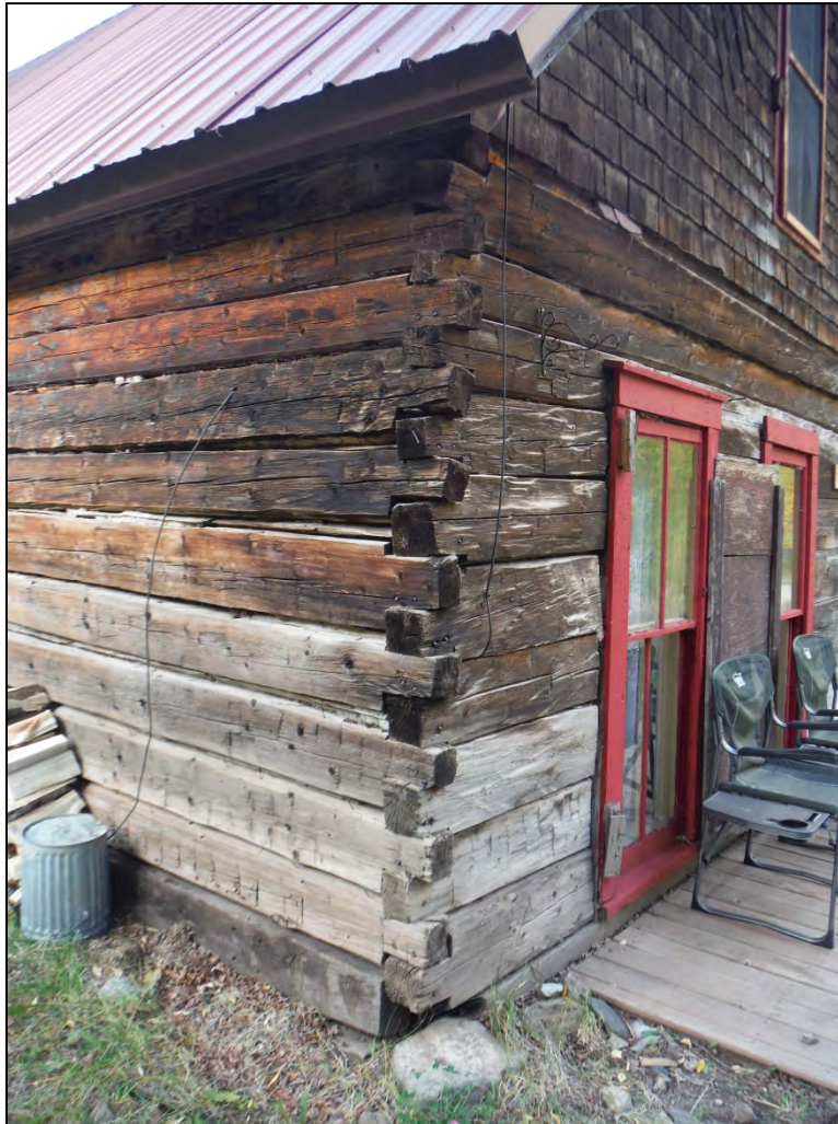
5GN6529 – Rosetta Cabin. Detail of square log notching on northeast corner. View southwest. (Roll 19-260, image 617, 09/27/2019)
