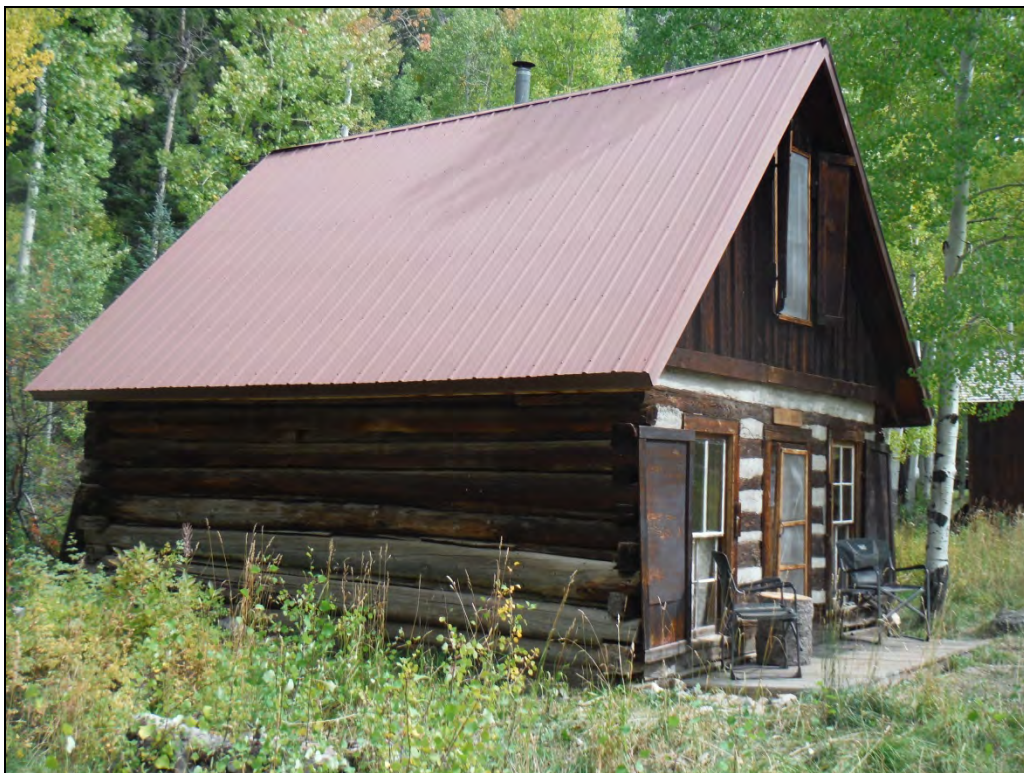
5GN6536 – Clayton Cabin. Oblique view of the southwest corner. View northeast. (Roll 19-259, image 515, 09/26/2019)
