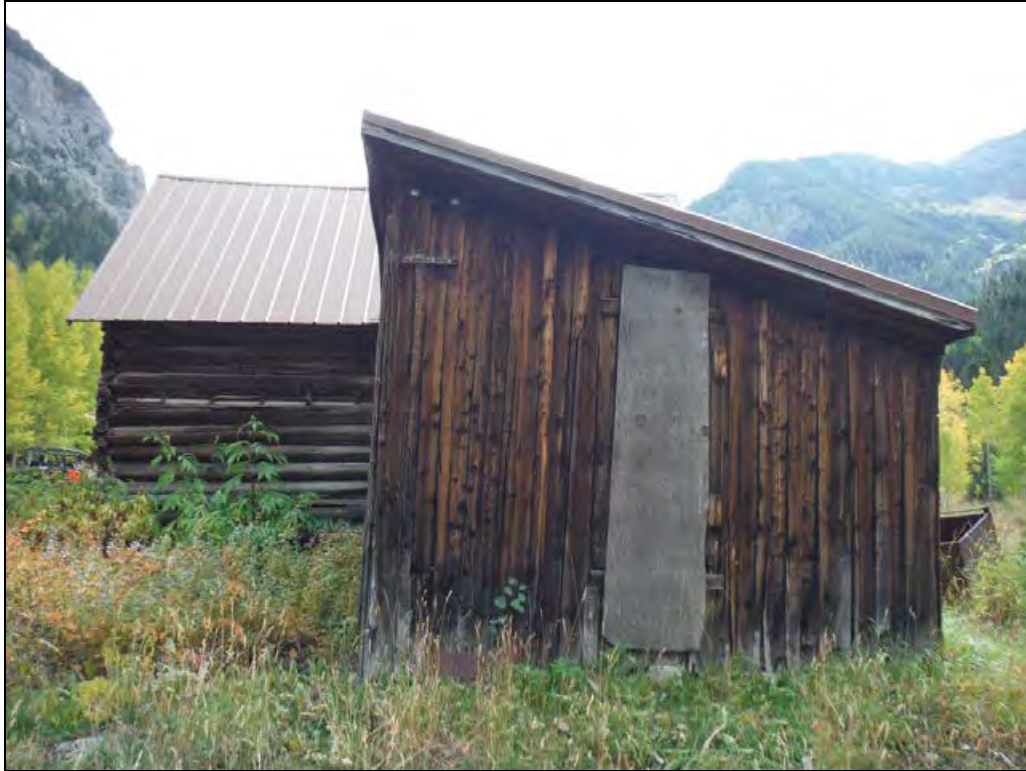
5GN6528 – General Store. View of west elevation. View east. (Roll 19-260, image 716, 09/27/2019)
