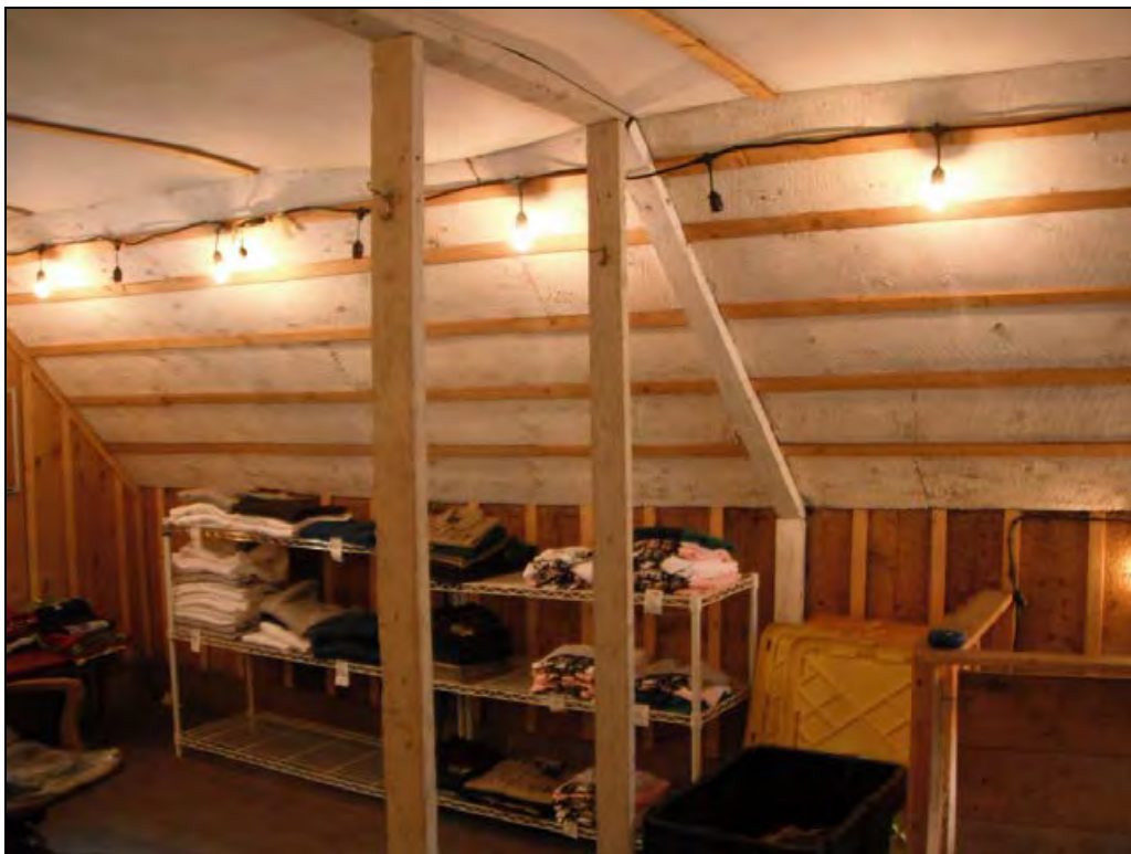
5GN6528 – General Store. View of the interior, ceiling and northeast corner/east wall on the second floor. View northeast. (Roll 19-261, image 240, 09/27/2019)
