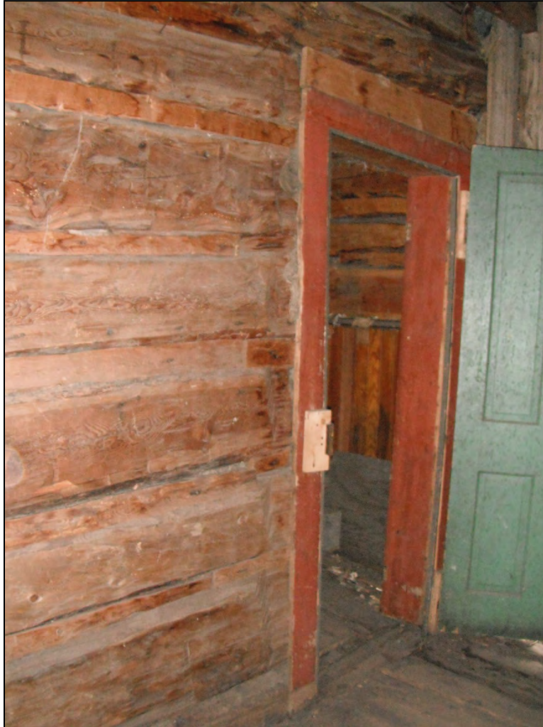
5GN6527 – Crystal Club. Interior, view of the door in the south wall of the original building which leads into the “front room” of the addition. The log wall photo left would have originally been exterior. View northeast. (Roll 19-262, image 266, 09/27/2019)
