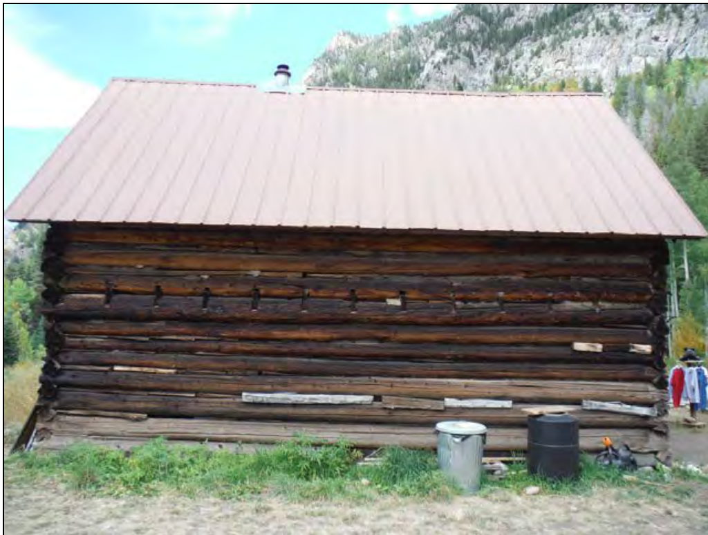
5GN6528 – General Store. View of east elevation. View west. (Roll 19-260, image 733, 09/27/2019)
