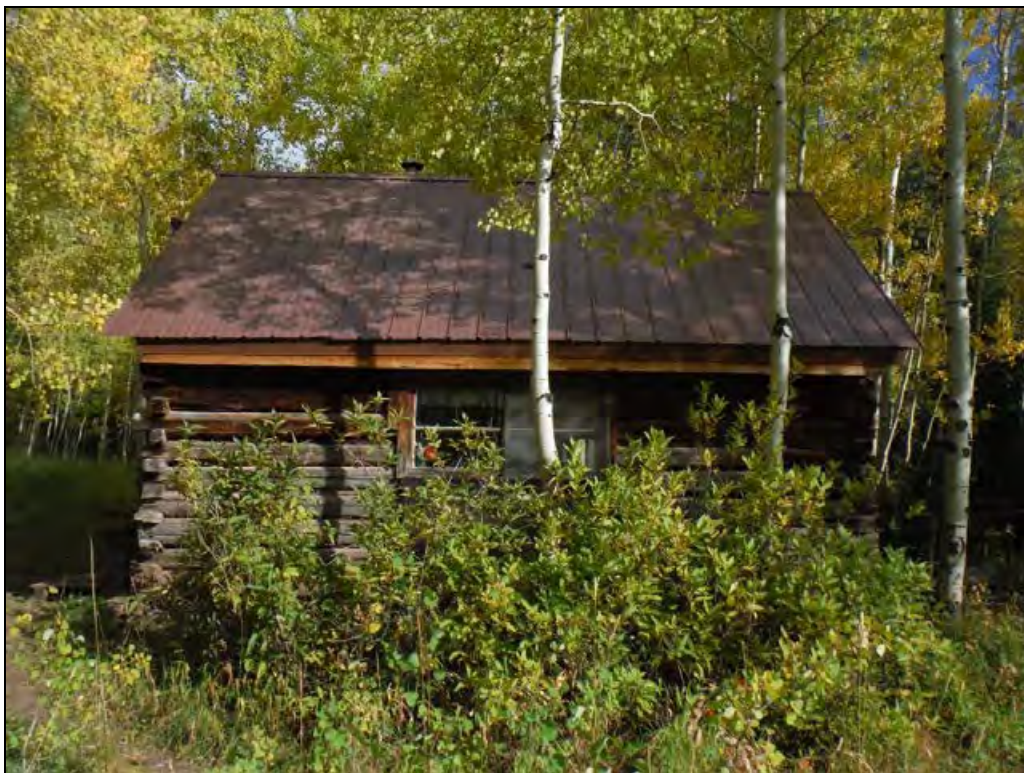
5GN6530 – Edgerton Cabin. View of west elevation. View east. (Roll 19-259, image 592, 09/26/2019)
