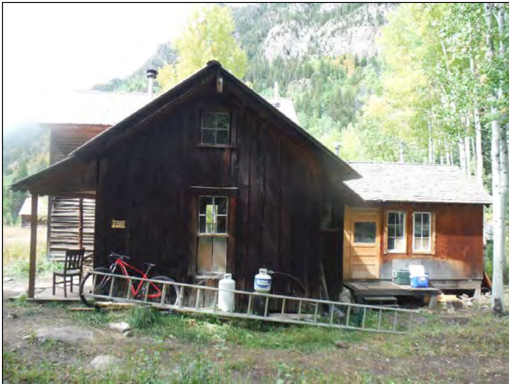
5GN6535 – Melton House. View of east elevation. View west. (Roll 19-259, image 521, 09/26/2019)
