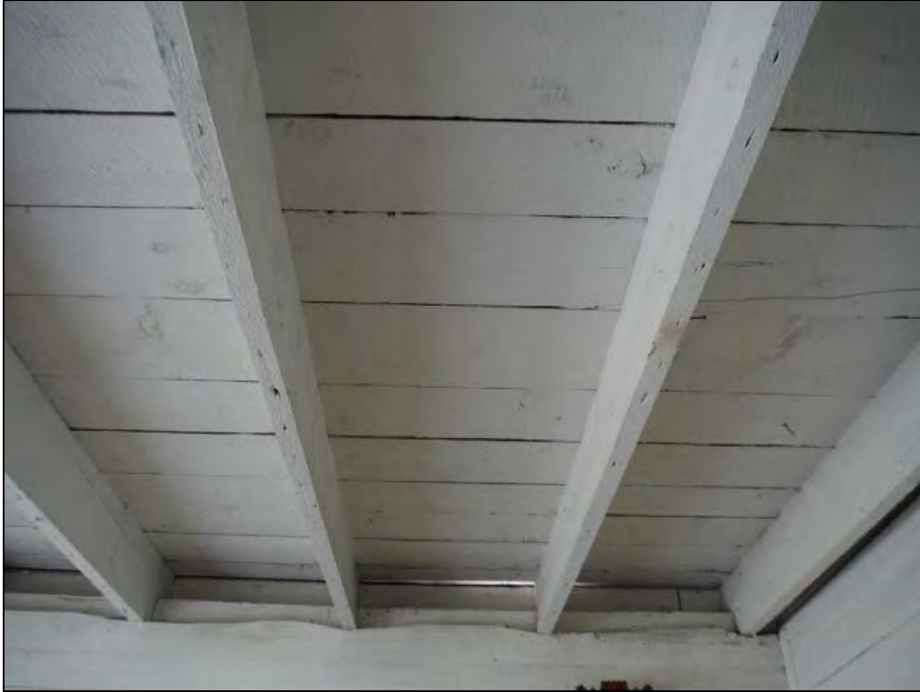
5GN6529 – Rosetta Cabin. Interior of the cabin, detail of the ground floor ceiling with floor joists and underside second floor floorboards visible. View up. (Roll 19-260, image 685, 09/27/2019)
