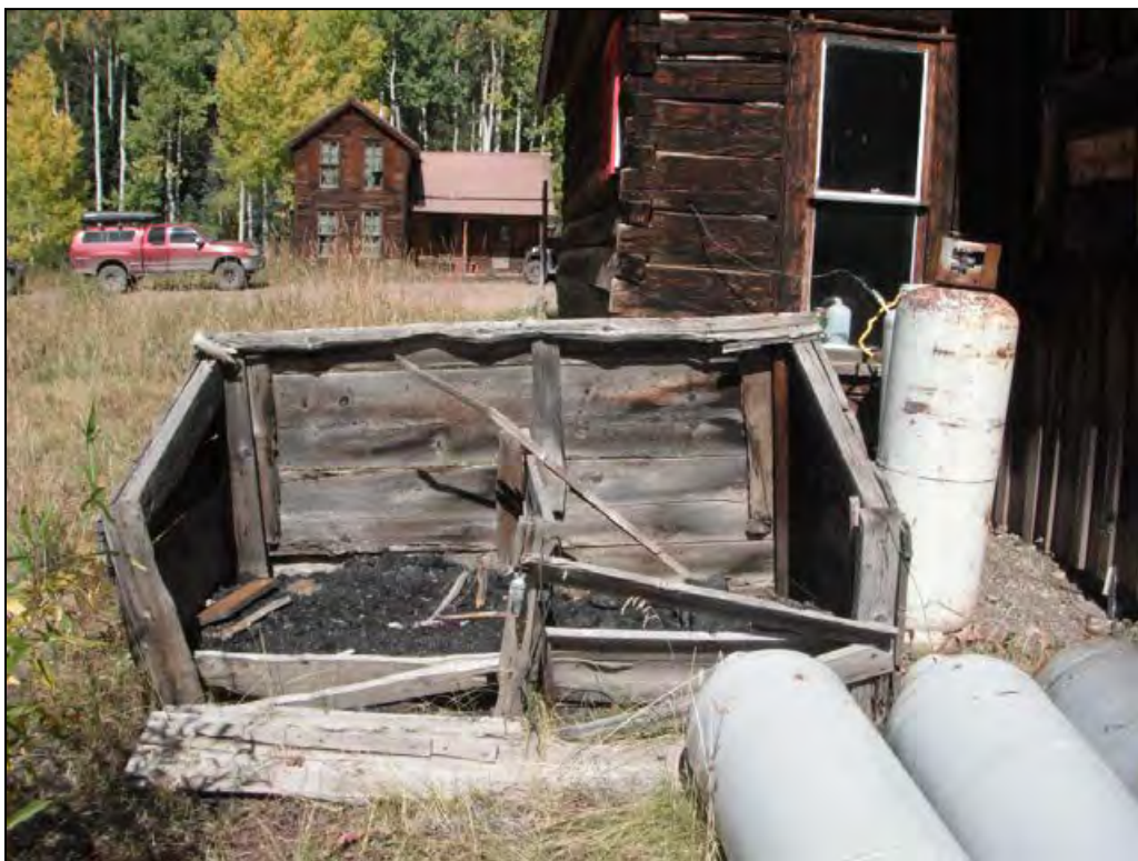
5GN6529 – Rosetta Cabin. View of coal bin located southwest of the cabin. View north. (Roll 19-261, image 186, 09/27/2019)
