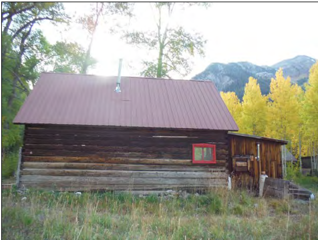
5GN6529 – Rosetta Cabin. View of west elevation. View east. (Roll 19-260, image 608, 09/27/2019)
