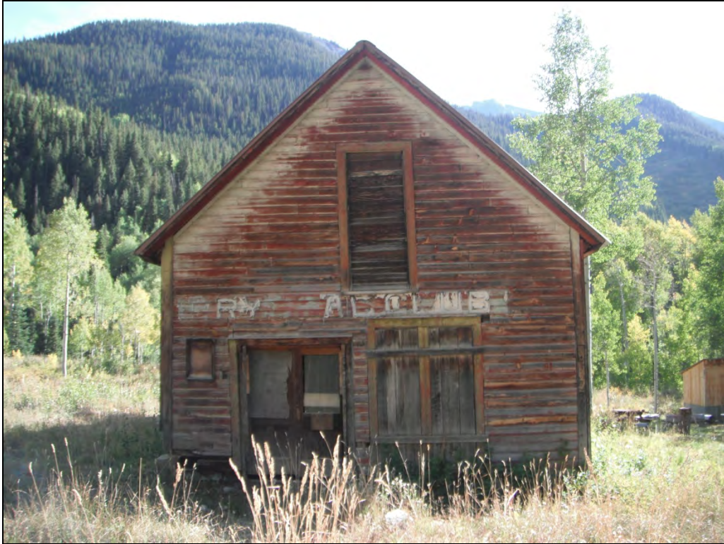
5GN6527 – Crystal Club. View of north elevation. View south. (Roll 19-258, image 65, 09/25/2019)
