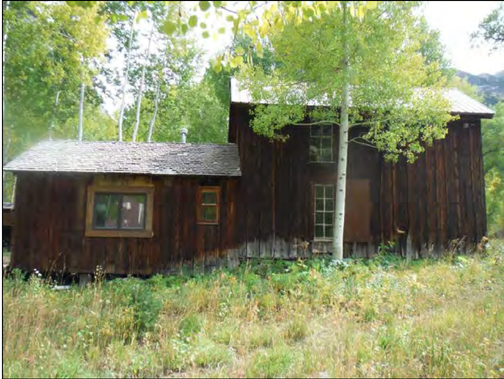
5GN6535 – Melton House. View of west elevation. View east. (Roll 19-259, image 526, 09/26/2019)
