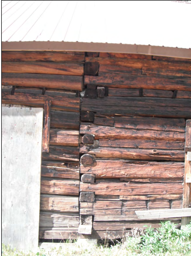
5GN6527 – Crystal Club. Detail of square log notching on the east elevation at the junction of the original building (photo right) and the historic addition (photo left). View west. (Roll 19-261, image 147, 09/27/2019)
