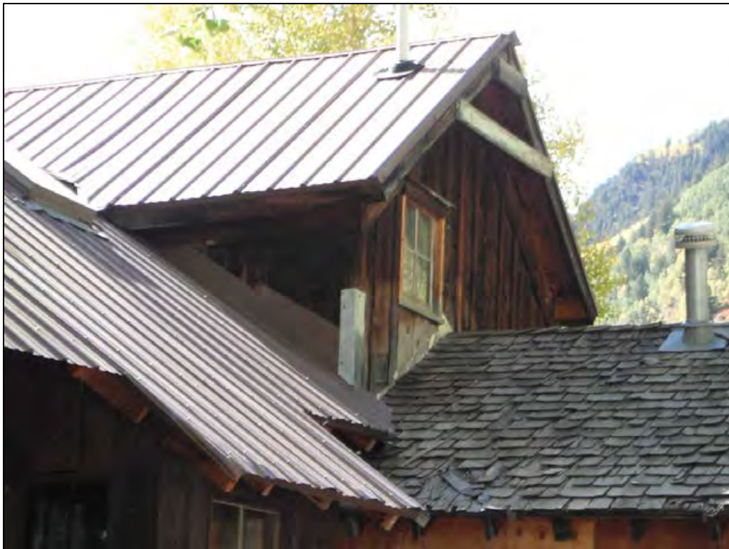
5GN6535 – Melton House. View of the gable on the north elevation of the original building also detailing shingles on the addition. View south-southwest. (Roll 19-261, image 208, 09/26/2019)
