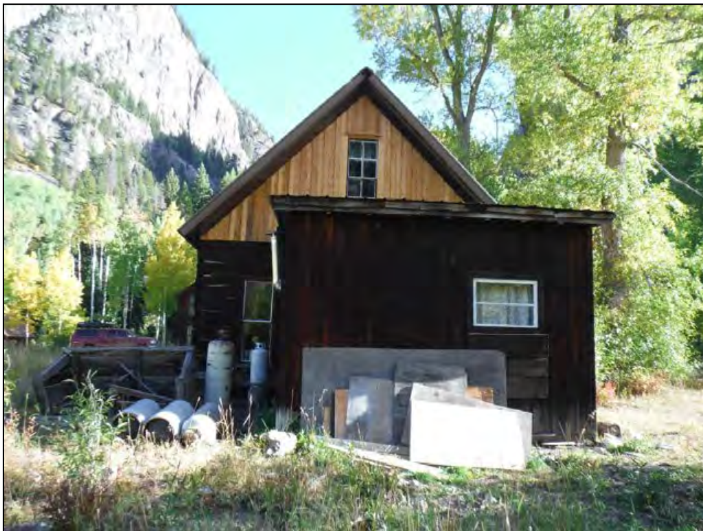
5GN6529 – Rosetta Cabin. View of south elevation. View north. (Roll 19-260, image 610, 09/27/2019)
