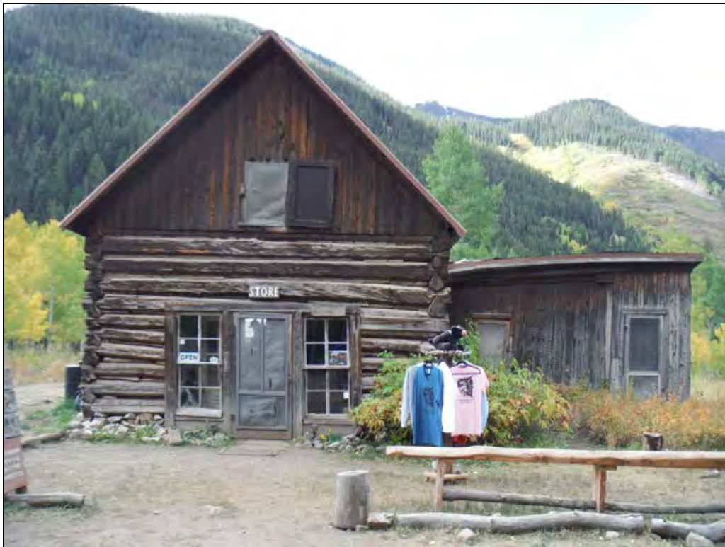
5GN6528 – General Store. View of north elevation. View south. (Roll 19-260, image 705, 09/27/2019)
