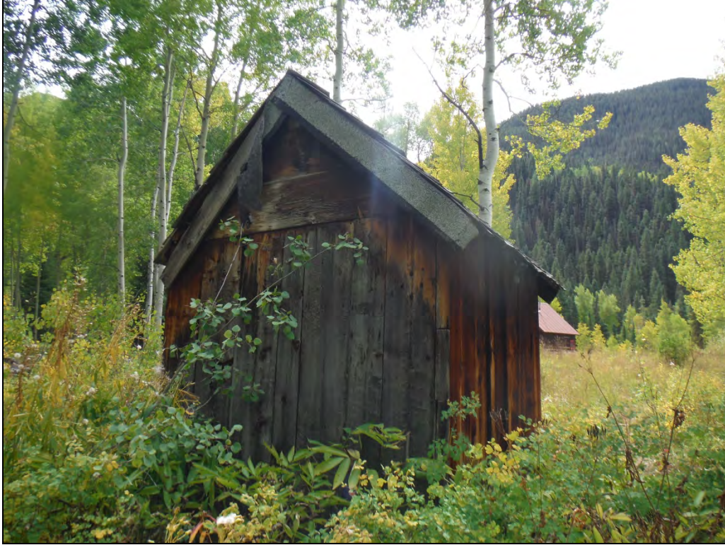
5GN6536 – Clayton Cabin. Oblique view of the northwest corner of the outhouse. View southeast. (Roll 19-259, image 516, 09/26/2019)
