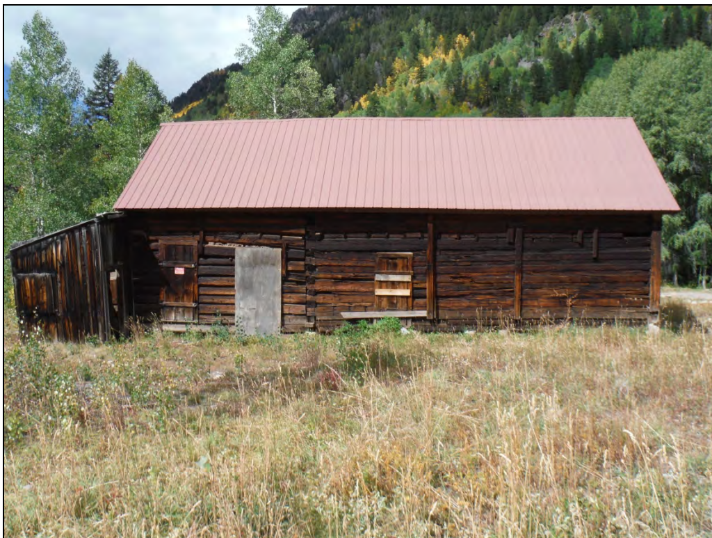
5GN6527 – Crystal Club. View of east elevation. View west. (Roll 19-260, image 742, 09/27/2019)
