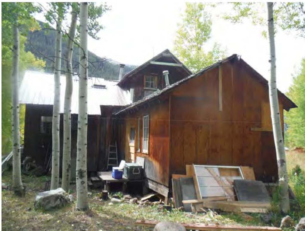
5GN6535 – Melton House. View of north elevation. View south. (Roll 19-259, image 524, 09/26/2019)
