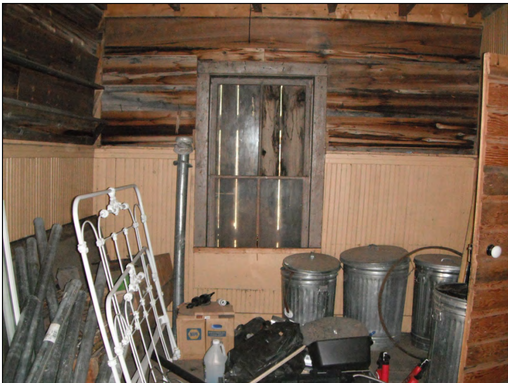
5GN6527 – Crystal Club. Interior, view of the west wall inside the back room of the addition. View west. (Roll 19-262, image 255, 09/27/2019)
