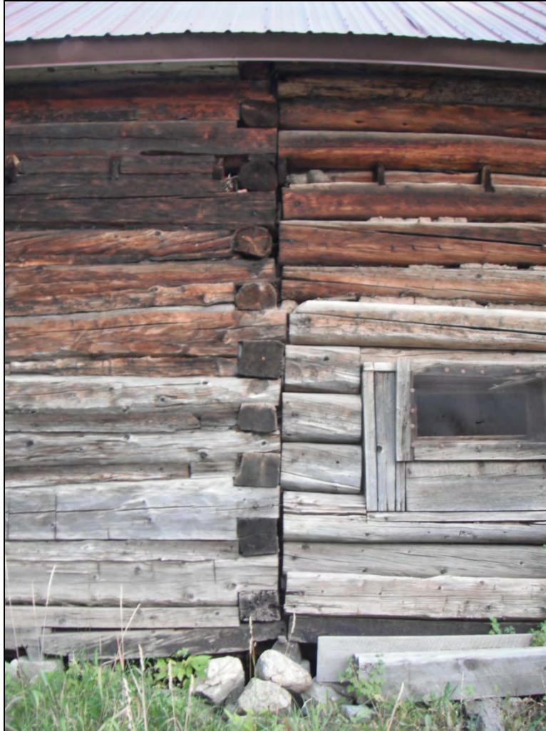
5GN6527 – Crystal Club. Detail of square log notching on the west elevation at the junction of the original building (photo left) and the historic addition (photo right). View east. (Roll 19-258, image 112, 09/25/2019)
