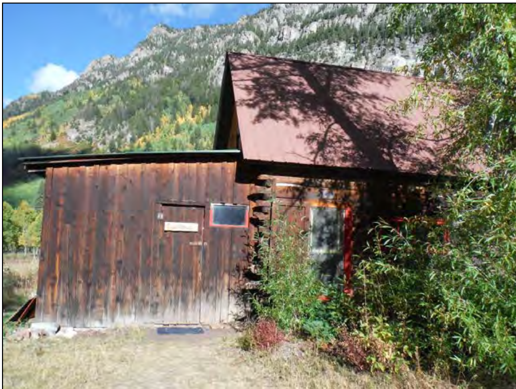
5GN6529 – Rosetta Cabin. View of east elevation including south end. View west. (Roll 19-260, image 613, 09/27/2019)
