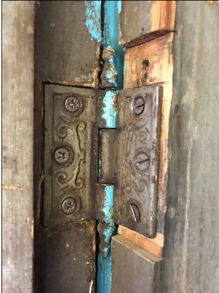
5GN6530 – Edgerton Cabin. Detail of decorative hinge on the front door (north elevation). View east. (Roll 19-261, image 131a, 09/27/2019)
