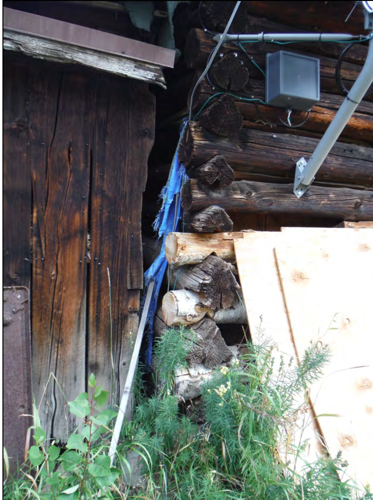
5GN6528 – General Store. Detail of steeply log notching on the southwest corner. View northeast. (Roll 19-260, image 725, 09/27/2019)
