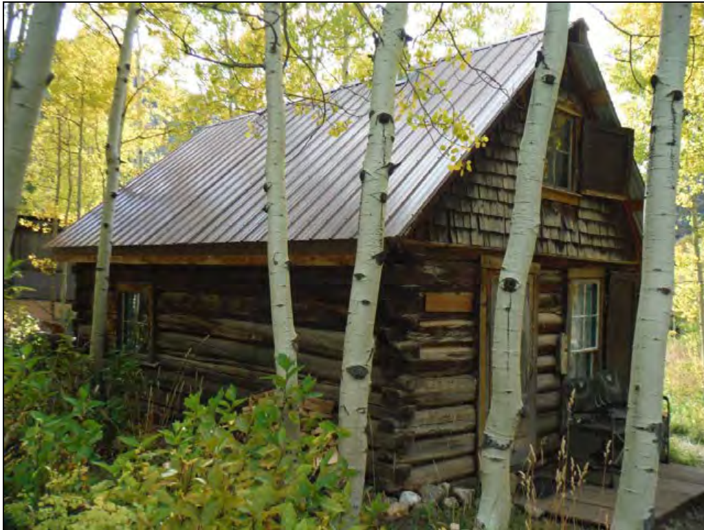
5GN6530 – Edgerton Cabin. Oblique view of northeast corner. View southwest. (Roll 19-259, image 599, 09/26/2019)
