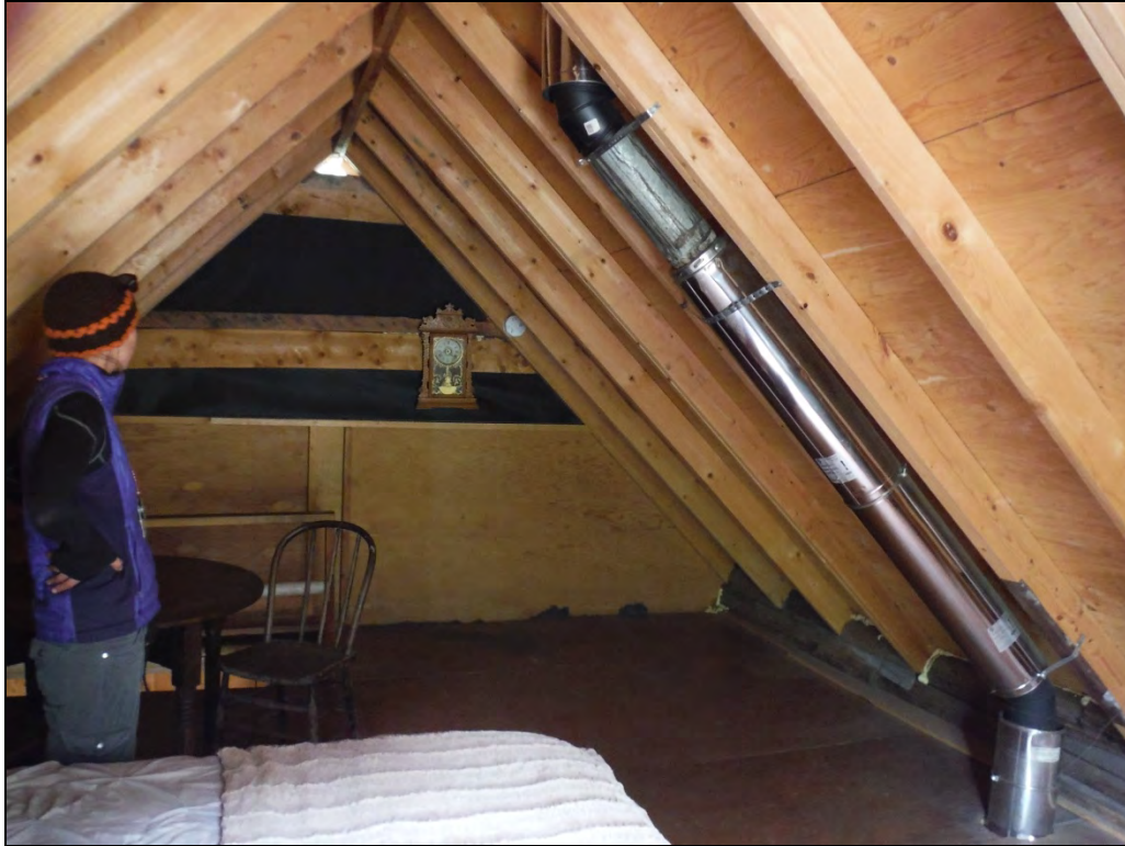
5GN6536 – Clayton Cabin. View of the interior of the cabin, second floor “attic” space. View north. (Roll 19-259, image 549, 09/26/2019)
