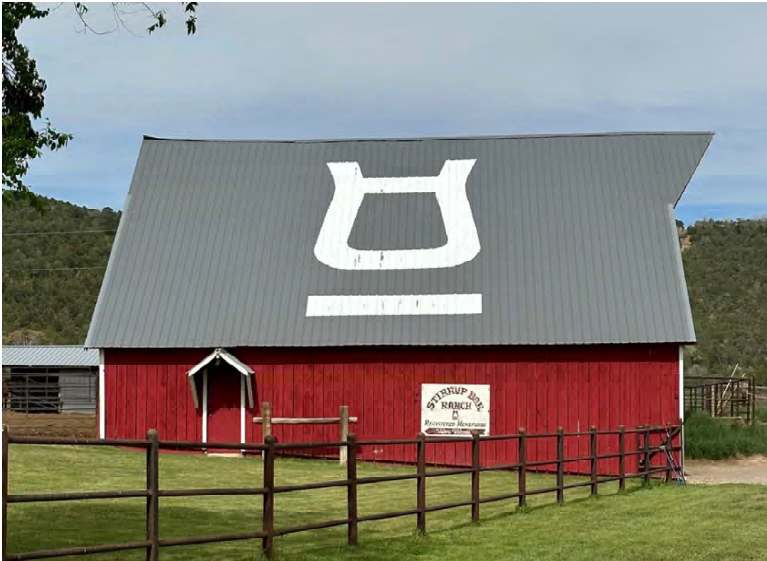
The Red Barn on the Headquarters Parcel's main entrance
