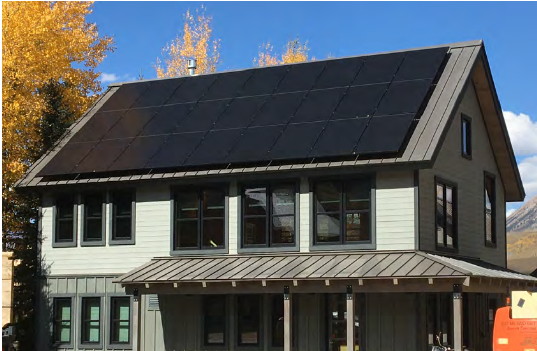
Residential Solar Installation in Crested Butte, CO 2020
